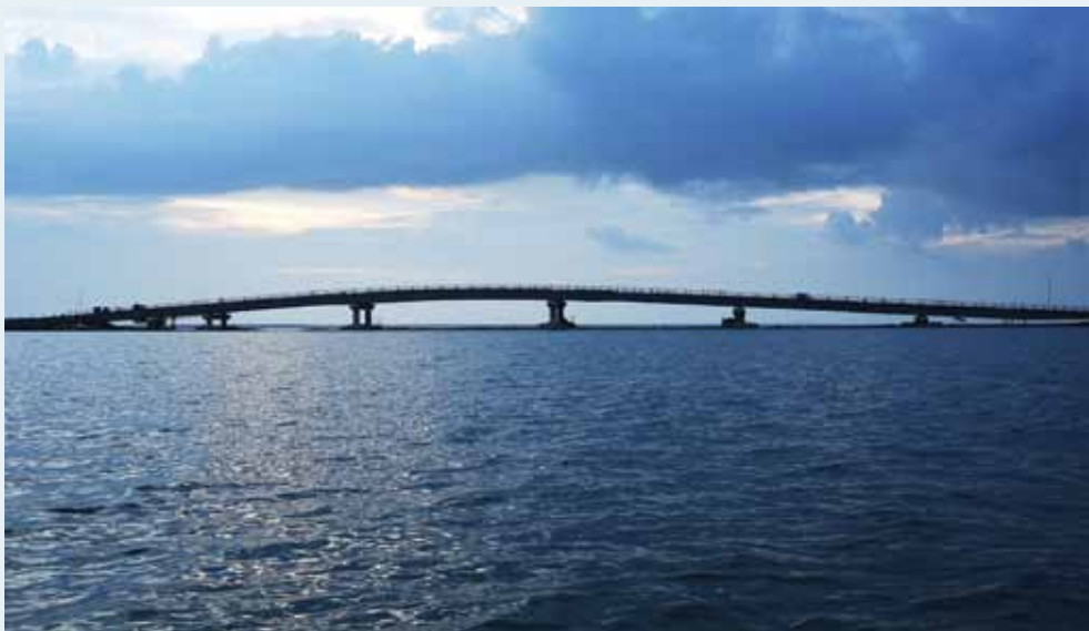
Sangupiddy Bridge across Kilali lagoon in Jaffna
