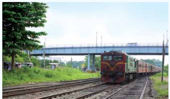
Completion of flyover across Veyangoda railway crossing
