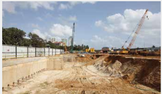
Commencement of foundation work at ITC Colombo One
