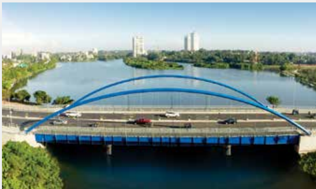
Completion of Polduwa Bridge across Diyawanna Oya
