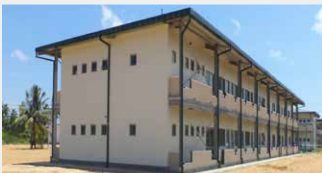
Completion of construction of prefabricated steel buildings at Lakvijaya Power Station
