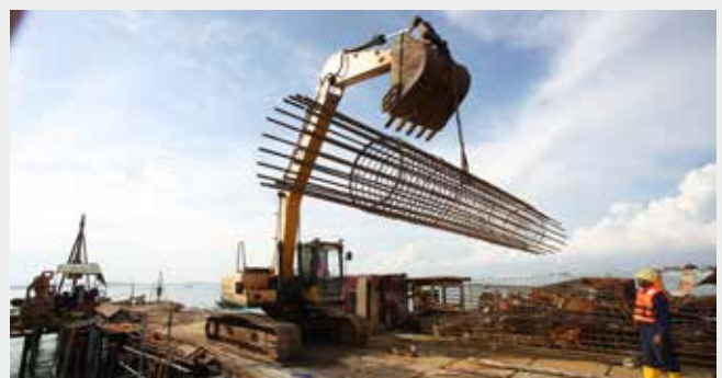
Commencement of construction of Kapparahota Jetty
