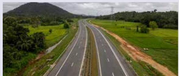
Completed the Central Expressway Project Package – A Stage 2 from Mirigama to Riloluwa
