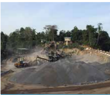
Commissioning of a new Crusher Plant in Mailapitiya
