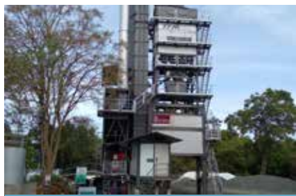
Commissioning of new Asphalt Mixing Plants in Ganewalpola, Thebuwana & Okewela
