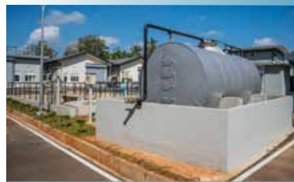
Completion of the Anuradhapura North Water Supply Project (Phase I)
