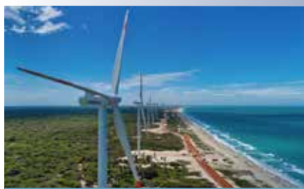
Completion of the Mannar Wind Power Project
