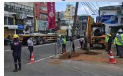
Commencement of construction of the Kohuwala Flyover under Hungarian financing
