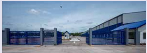
Construction of Sri Lanka's largest single roof warehouse
