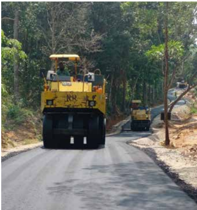
Use of carbon black modified asphalt in road works
