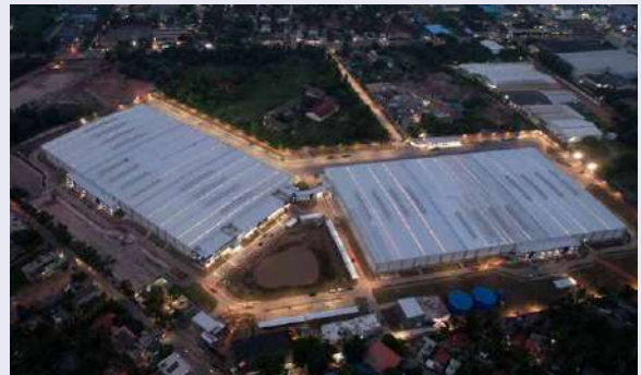
Substantial Completion of the Construction Work of Export Green Field Facility at Ekala (EGF2)
