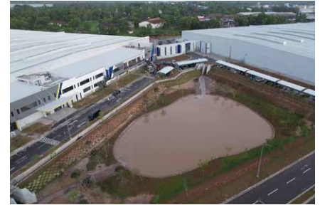
EGF Drain Control System
