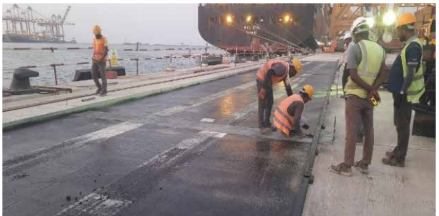
Specialised Asphalt mix containing Polymer Modified Bitumen (PMB) at Jaya Container Terminal
