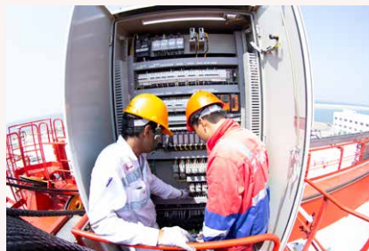
Repair of Port Machinery
